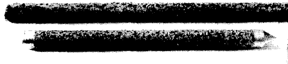
c) Slag deposits on recuperator tubes.
